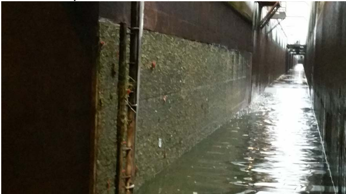
Figure 1. View of obscured side dewatering screen from floor of the Juvenile Collection Channel at McNary Dam on November 29, 2016.
