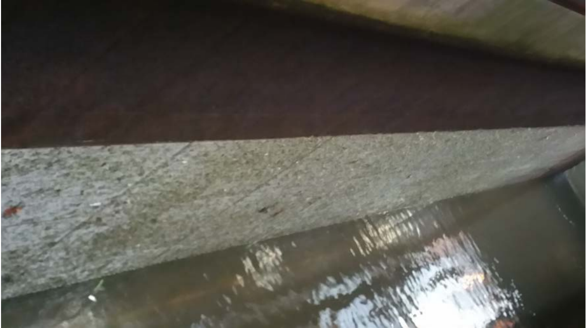
Figure 2. View of obscured side dewatering screen from access walkway, Juvenile Collection Channel at McNary Dam on November 29, 2016.
